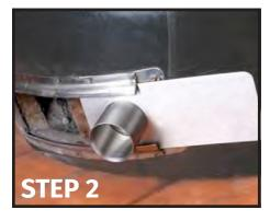
As you slide the Adaptor Door in, the light gauge stainless steel sheet metal will easily conform to the track.
