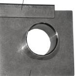
Place Expansion Clip like this for damper slide doors sized 2 3/4" to 3 1/4".
